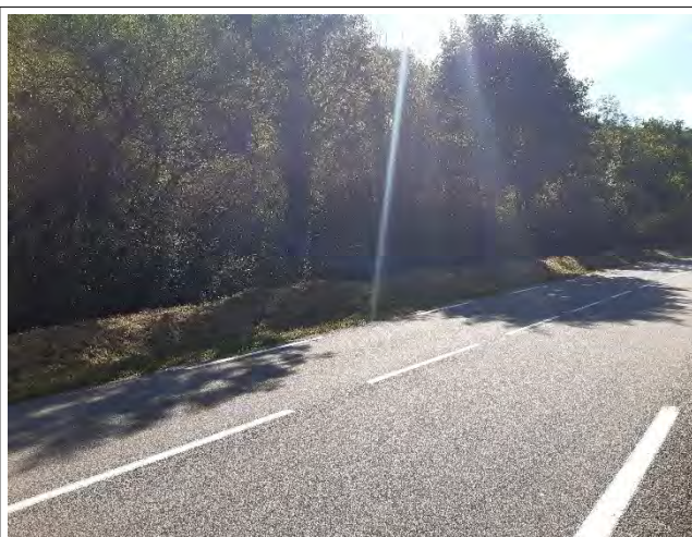
Merlon longeant la RD904
